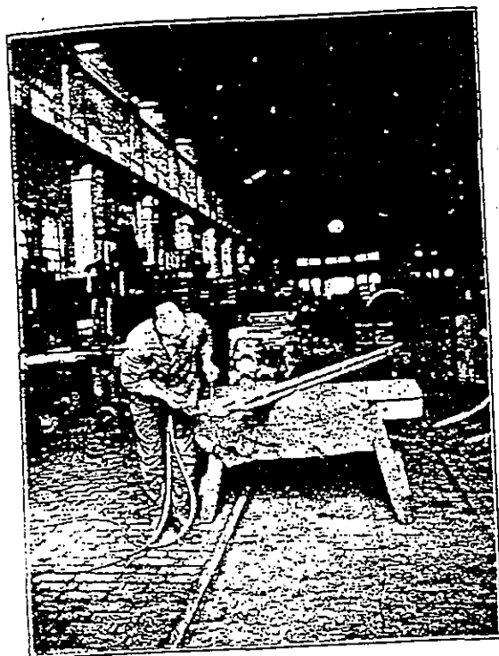
Oxy-Acetylene Welding Superheater Elements.
